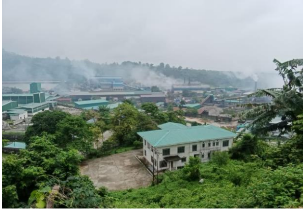
Figure 29: Pasakha Industrial Estate at a glance
