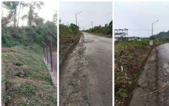
1. Clearing of grass - Completed
