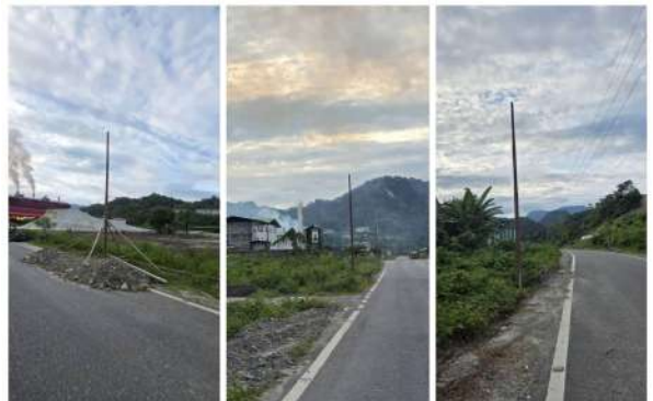
2. Maintenance of Streetlights - completed
