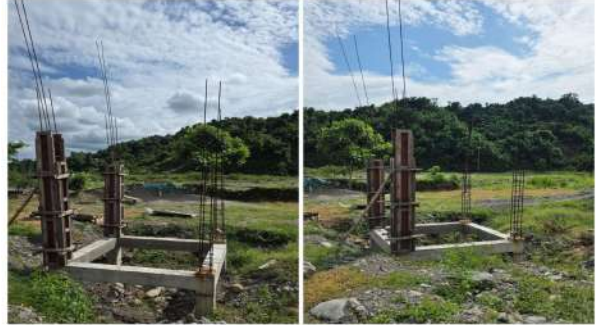
6. Construction of Watchtower - Work Ongoing (Physical Progress less than 5%, Financial Progress 3%)
