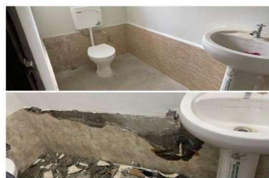
4. Toilet facility leakage remediation
