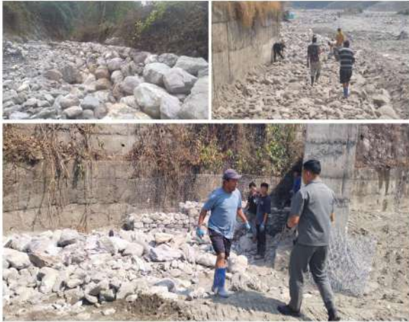
5. Construction of Flood protection measures along Singyechu - Completed
