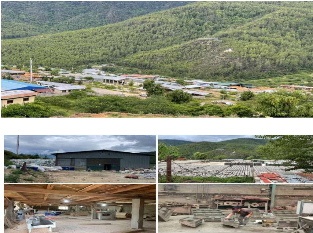
Figure 26: Bjemina Industrial Estate
