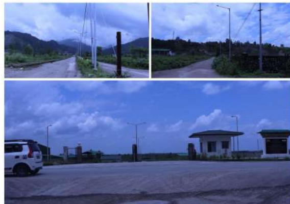
2. Maintenance of Streetlights - completed
