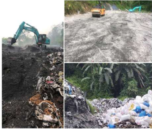
6. Levelling of Waste - Completed
