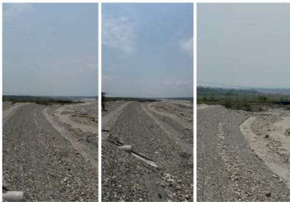
1. River Training Works (DIP) - 92% completed
