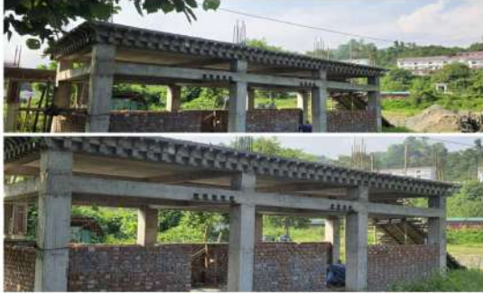
5. Construction of Public toilet - Work Ongoing (Physical Progress 52%, Financial Progress 40%)
