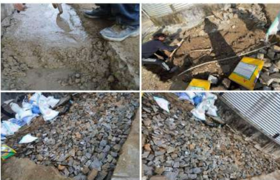
3. Concrete restoration adjacent to reservoir tanks
